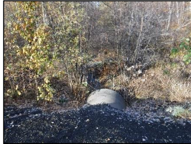
Figure 6.57: Culvert at Arlington Boulevard
