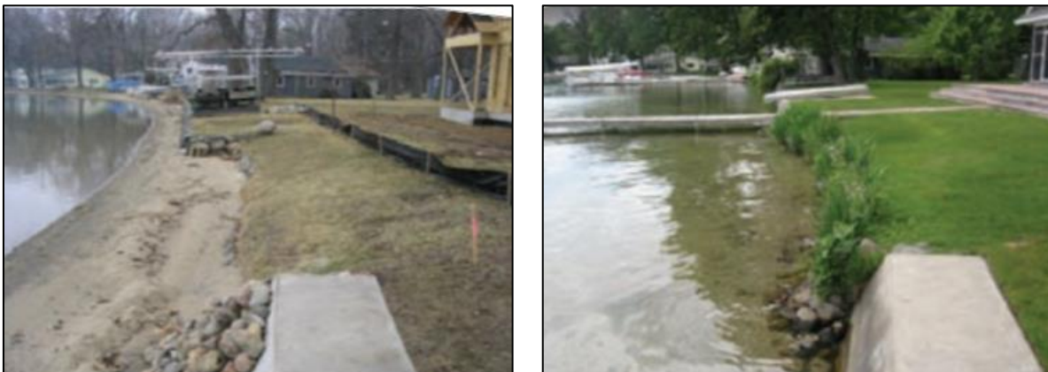
Figure 6.19: A typical lake shoreline before (left) and after (right) bioengineering to protect it from wave action
