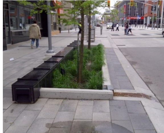
Figure 6.5: Bioretention Planter
