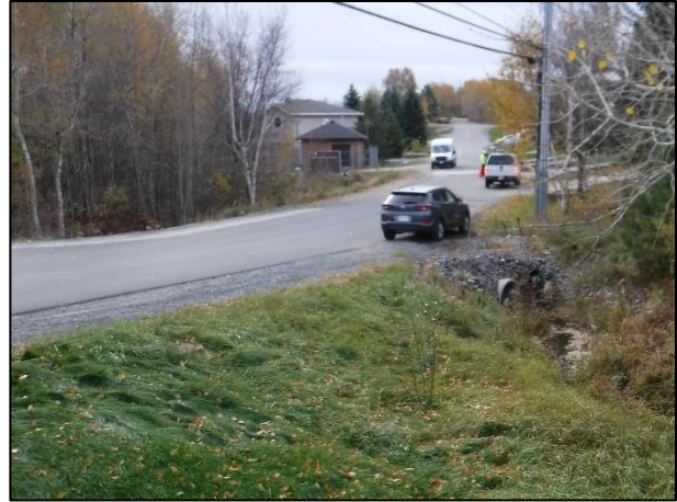
Figure 6.54: Culvert at 4 th Ave, showing road
