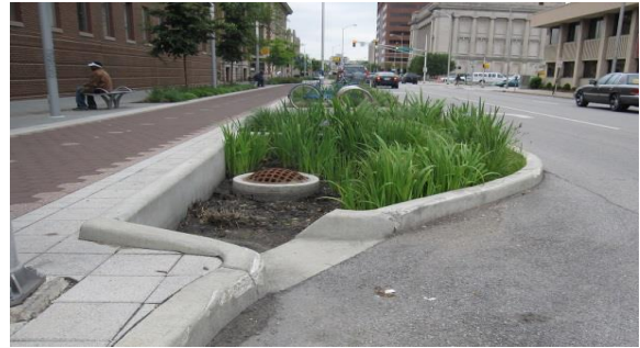
Figure 6.3: Bioretention Bump Out
