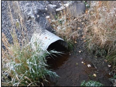
Figure 6.56: Culvert at South Bay Road
