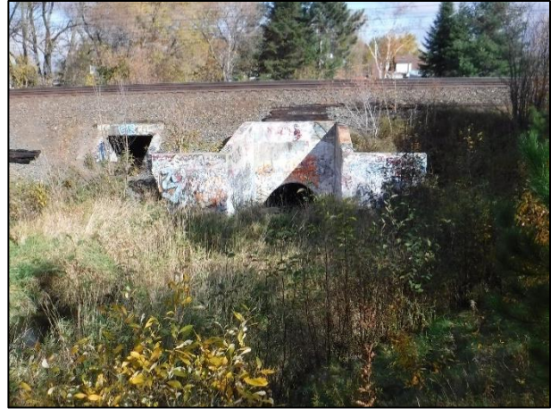
Figure 6.49: Storm sewer outlet downstream of railway
