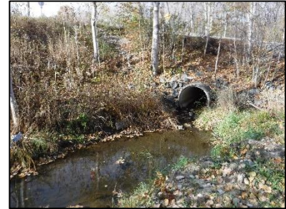
Figure 6.58: Culvert at Keast Drive
