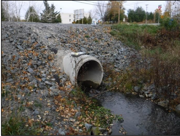
Figure 6.53: Culvert inlet at 4 th Ave.
