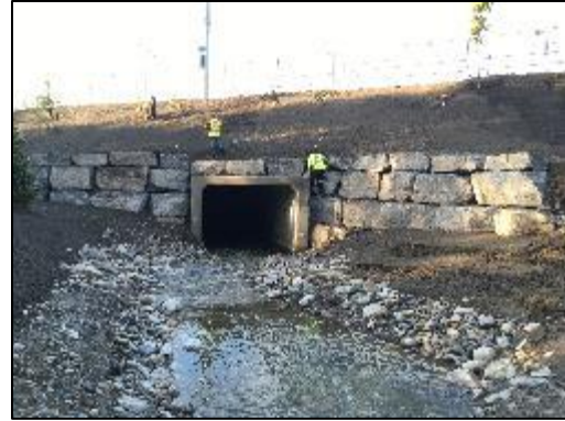
Armourstone retaining wall for culvert inlet protection and road embankment support
