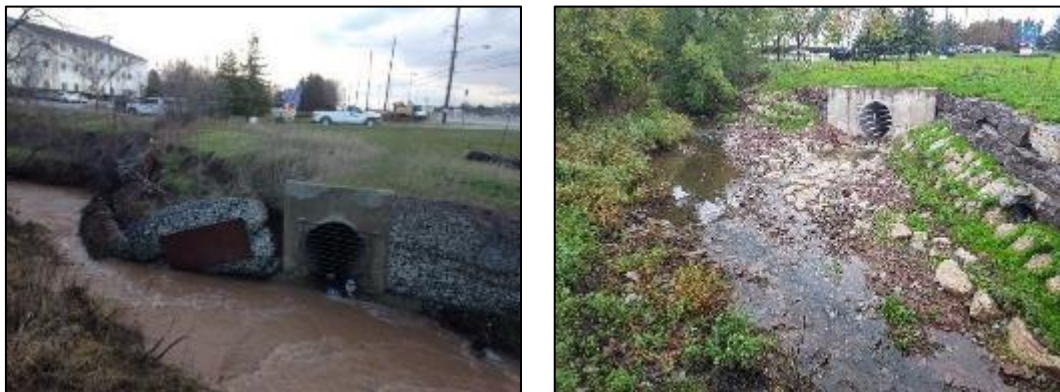
Figure 6.26: Before and after example of local bank works
