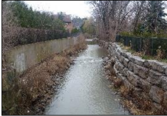
Armourstone retaining wall and concrete floodwall
