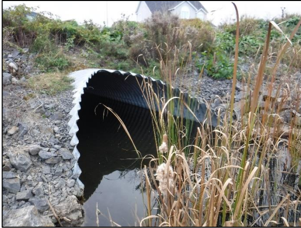
Figure 6.45: Inlet to the Greenwood Drive culvert
