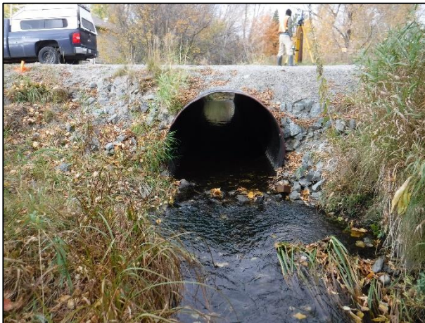
Figure 6.50: Culvert outlet at Rita St.
