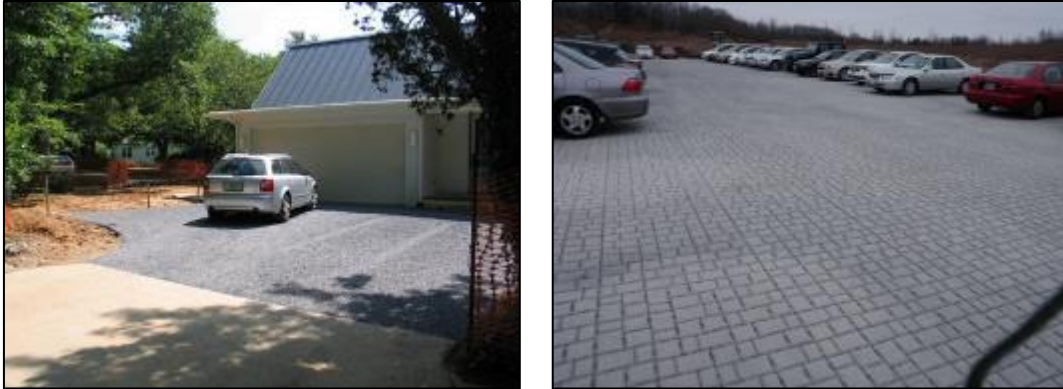
Figure 6.17: Typical Permeable pavement on residential and commercial properties
