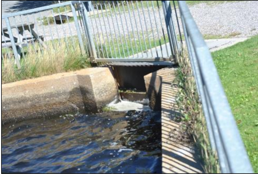
Figure 3.63. Water Control Structure, Outflow of Lake Laurentian.
