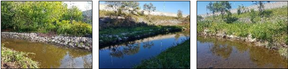
Immediately after construction
