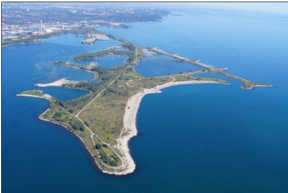
Figure 9.15: Aerial view of Tommy Thompson Park, Toronto, Ontario, Canada.
