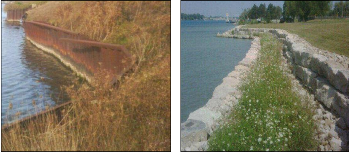
Figure 6.20: Before and after showing a shoreline improved with a rocky revetment, incorporating biodiversity (from St. Clair River shoreline restoration report, 2014 [ https://www.friendsofstclair.ca/www/pdf/resources/2014/Shoreline%20Restoration%20report.pdf ])
