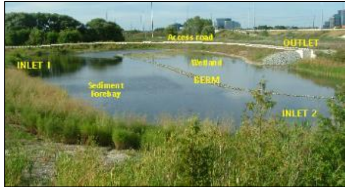
Figure 6.10: Components of a wet stormwater management facility.
