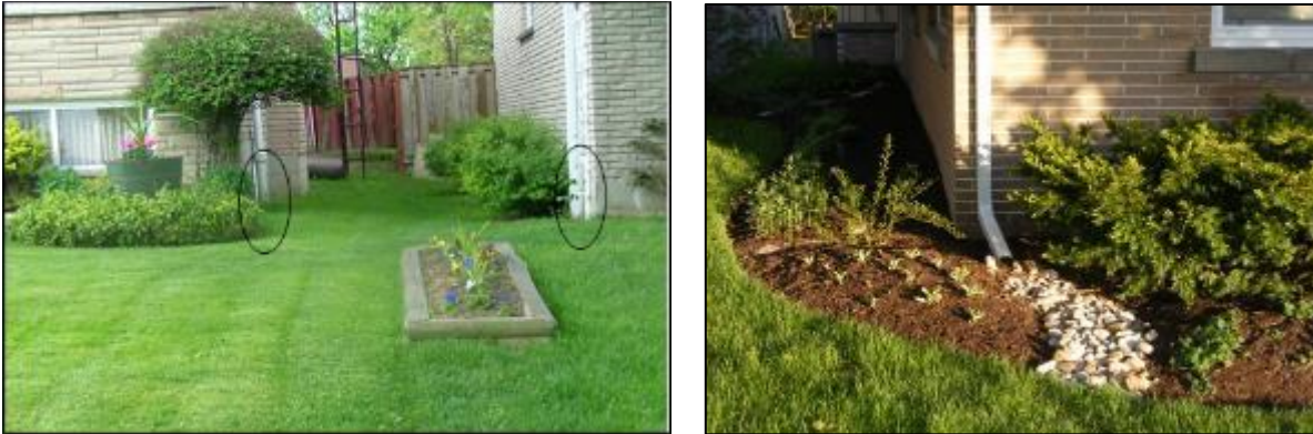
Figure 6.14: Example of downspout disconnection.
