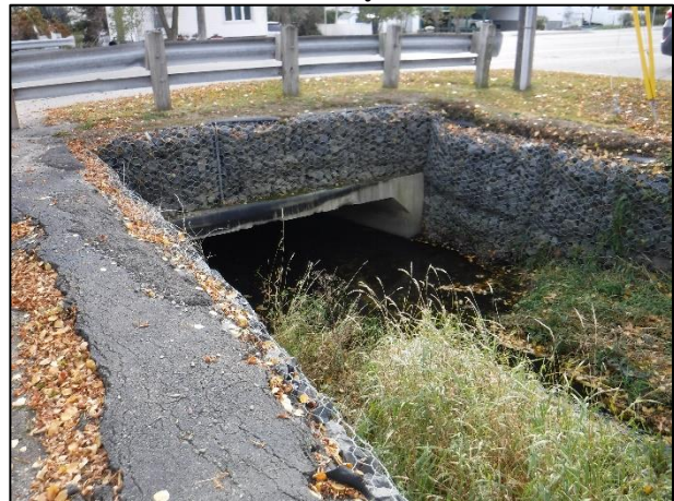
Figure 6.51: Culvert inlet at Bancroft Dr.
