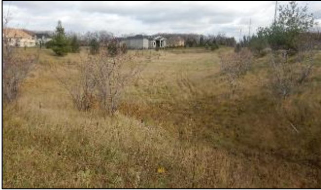
Figure 6.11: A dry stormwater management facility
