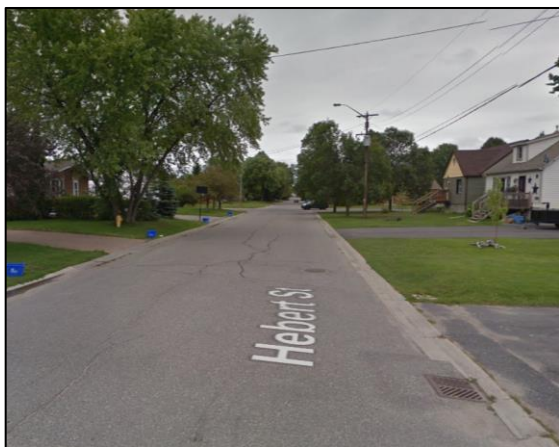
Figure 6.29: Example of an urban cross section (curb & gutter) along Hebert Street in Sudbury (source: GoogleEarth)
