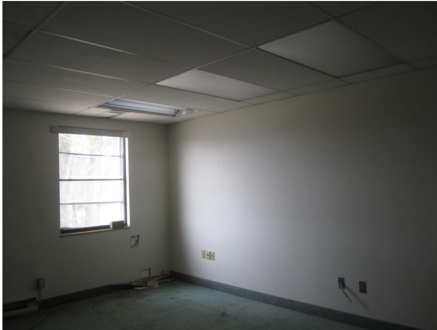
Photograph No. 5. Lead containing cream coloured paint found throughout main floor and typical acoustic ceiling tiles.
