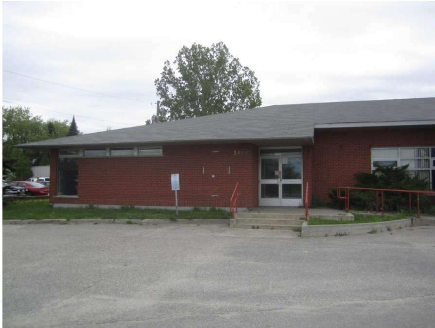
Photograph No. 1. Site property and building at 3400 Highway 144, Chelmsford, Ontario.
