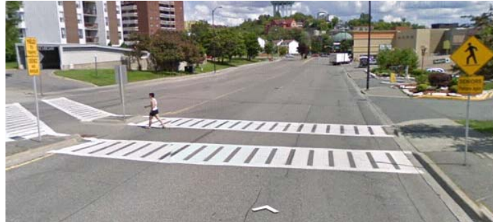
Improved Ste Anne's Road crossing
