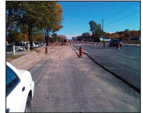
Municipal Road 80, Hanmer (Frost Avenue to Glenn Street)
