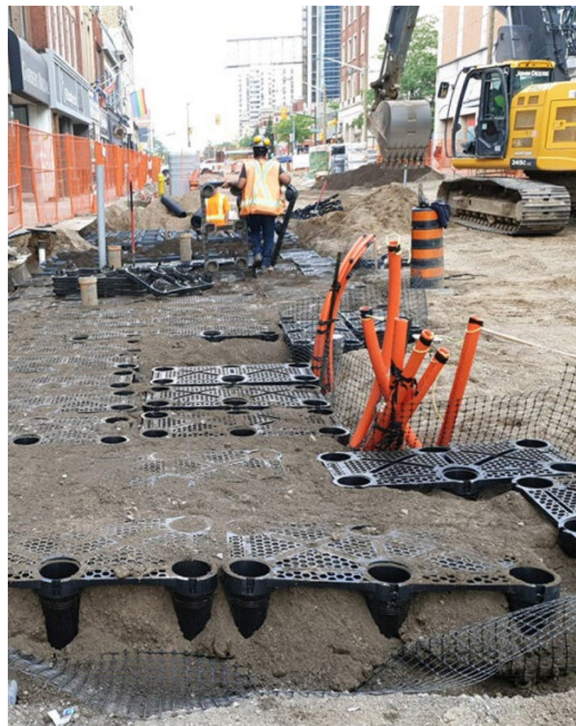
Image 13 – Underground plant cells installation for mature canopy trees, Dundas Place, London, Ontario. Credit: Dillon Consulting.
