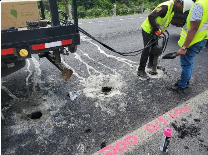
Photo 2: Wet, malleable asphalt/underlying material from the 5 th set of cores.
