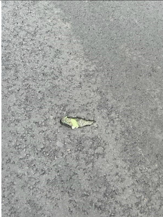
Photo 7: Plastic bottle observed in the surficial asphalt near STA 2+000.
