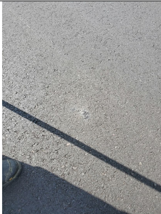
Photo 4: Moderate segregation at Section 8.
