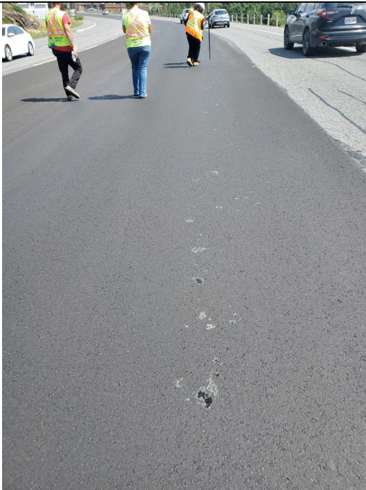
Photo 11: Fat spots observed at Survey Points 124 and 125.
