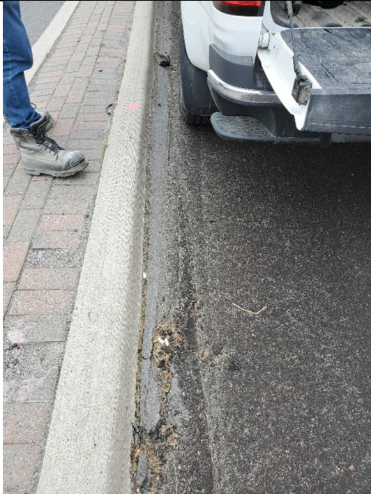
Photo 5: Cracks/loose asphalt observed in the section along the centre island.
