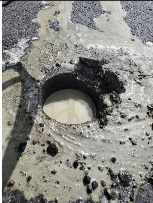
Photo 6: Core 5A hole with lifted/fractured edges.
