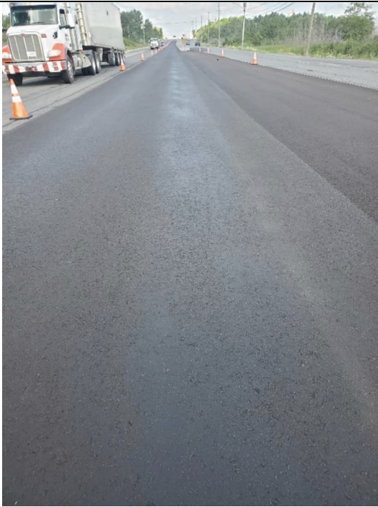
Photo 5: Flushing observed in Section 10.
