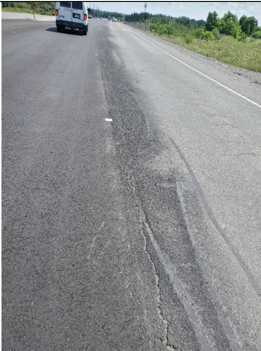
Photo 9: Burned asphalt at Survey Points 100 and 101.
