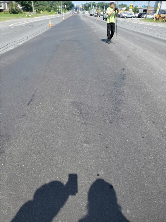
Photo 7: Hydraulic oil contamination at Survey Point 68-69.
