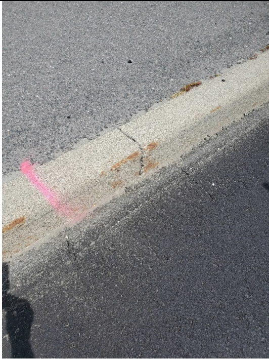
Photo 5: Cracks observed in the asphalt along the centre island.
