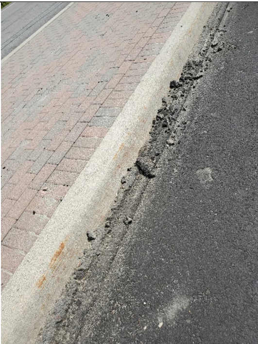
Photo 3: Broken/loose older existing asphalt in thin strip along the eastbound passing lane centre island.
