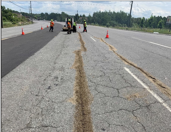
Photo 1: RSR preheating the road surface along the Kingsway.
