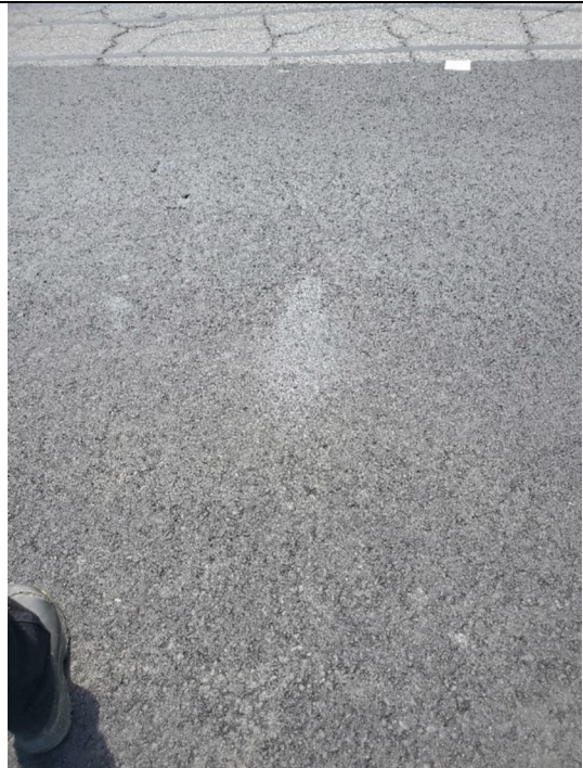
Photo 8: Fat spot observed at Survey Point 93.
