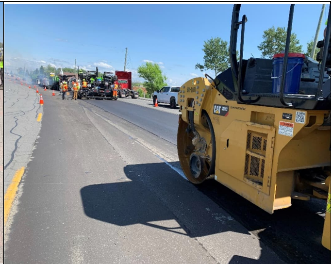
Photo 6: compacting the asphalt lift with a smooth-drum roller (12 T).
