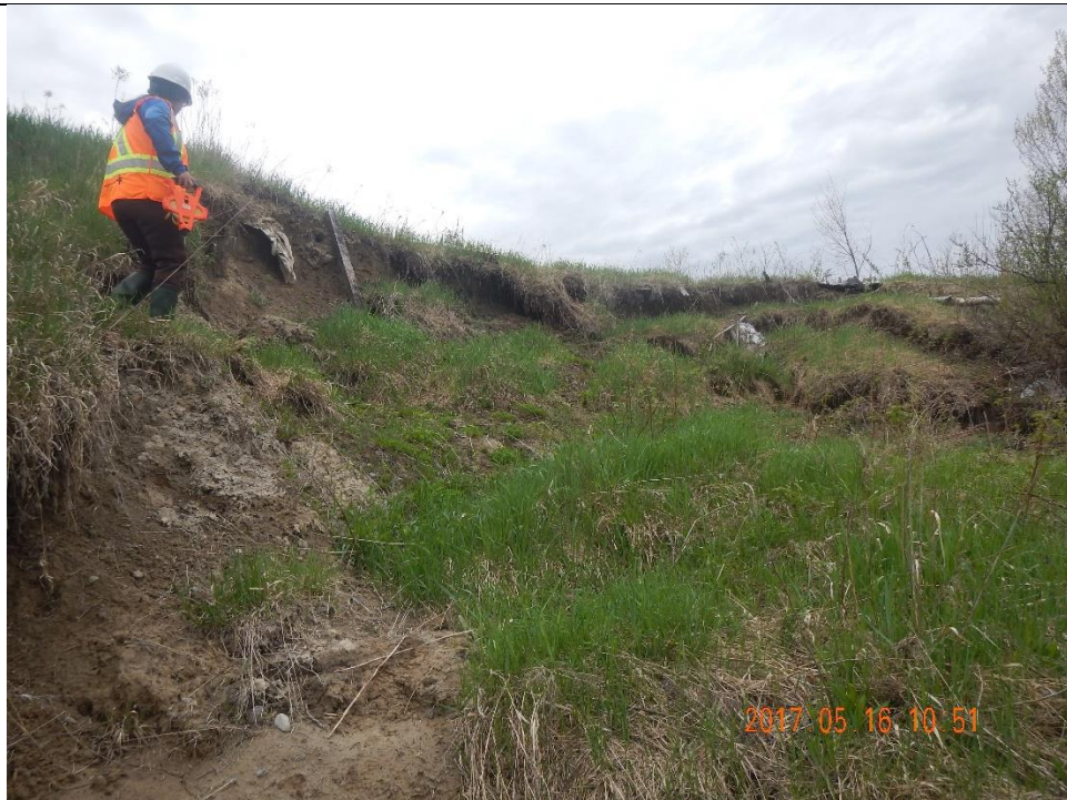
Photograph taken facing left bank. Large erosion scar observed.
