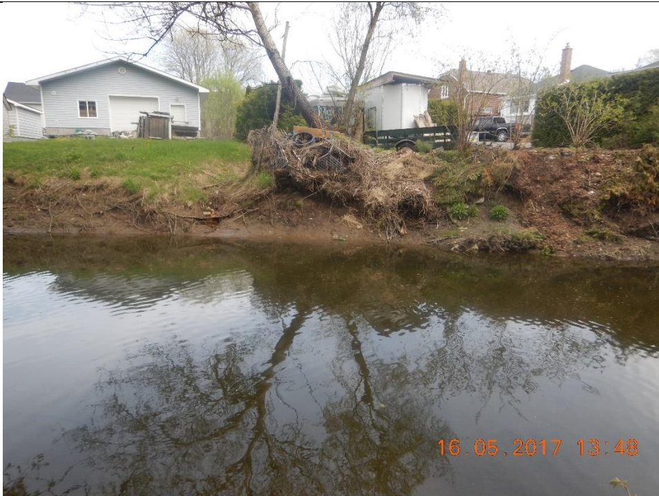
Photograph taken facing left bank. Bank failure present and trash line observed at property edge.
