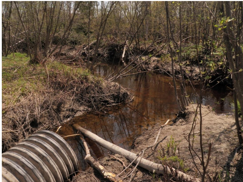
Photograph taken facing downstream toward right bank. Pipe outlets common throughout reach. Failure and erosion of right bank observed.
