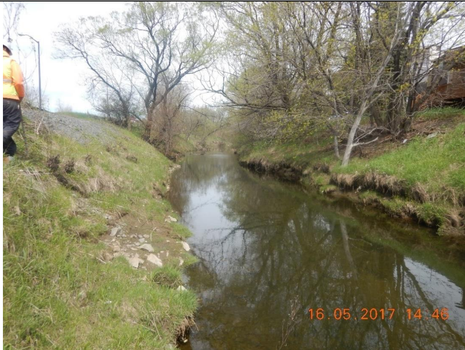
Photograph taken facing upstream. Undercutting, slumping, and pipe outlets common. Rip rap observed.
