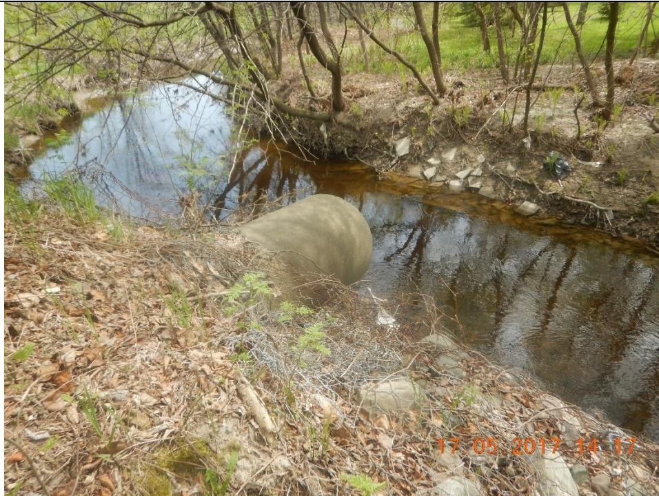
Photograph taken facing upstream. Exposed tree roots and rip rap observed. Pipe outlets undercutting banks were common.
