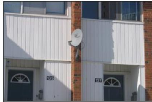
Fastened to Brick Wall Outside Unit
