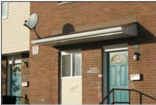
Fastened through Roofing
