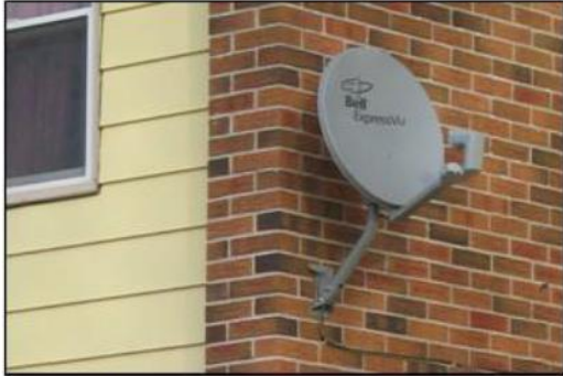
Fastened to Brick Wall Outside Unit
