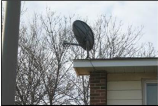
Fastened through Roofing
