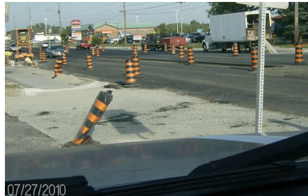
Inferior Asphalt Removed Next Day
