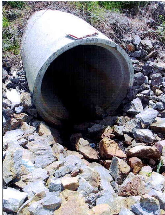
Plate 8: Creek culvert at The Kingsway showing low flows
