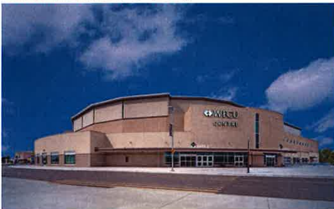
Figure 26 WFCU Centre, Windsor ON (2008)
