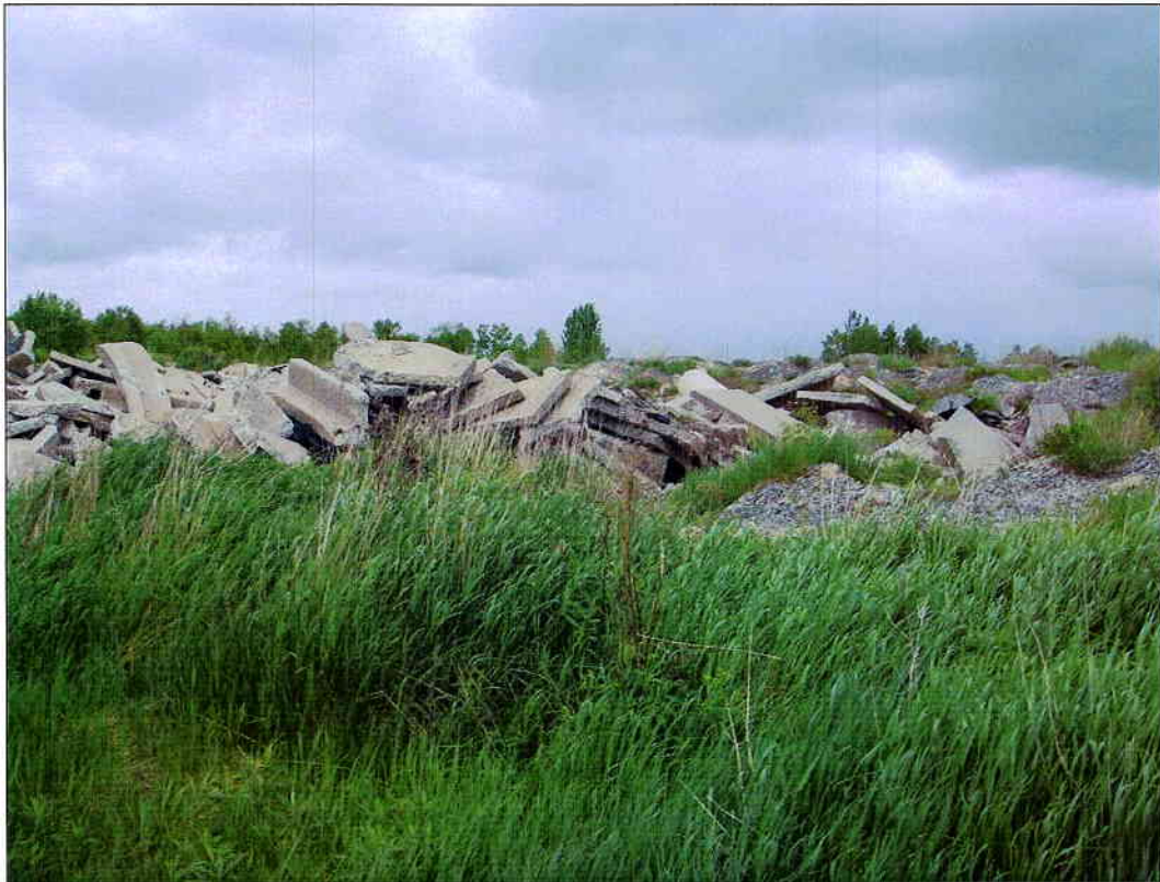
Plate 2: Demolition waste materials located in south-east corner of site
