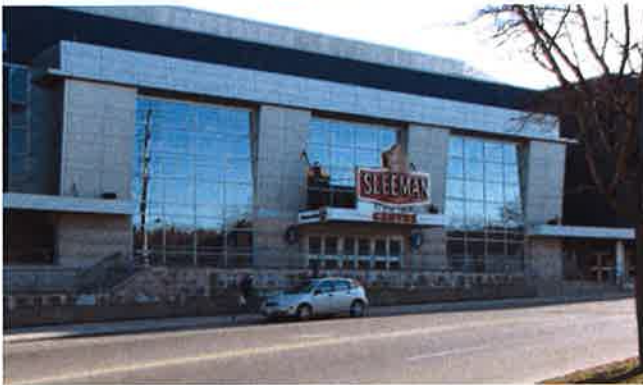
Figure 22 Sleeman Centre, Guelph ON (2000)
