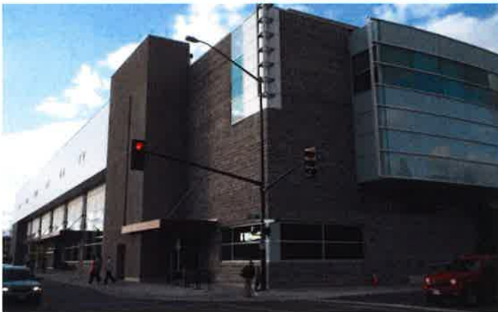
Figure 25 Rogers K-Rock Centre, Kingston ON (2008)
