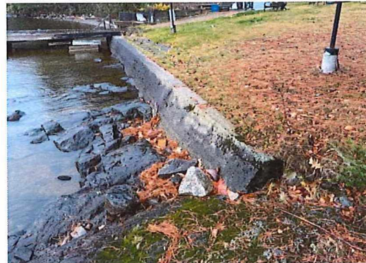
Photo 4. Breakwall on bedrock substrate
