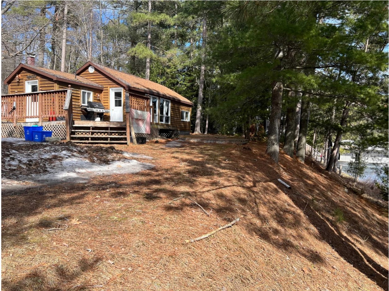
Photo 1: Existing building on upper plateau showing no signs of slope instability.
