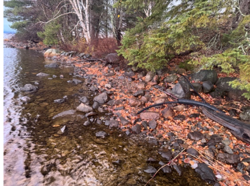
Photo 2. Boulder toe at base of bluff
