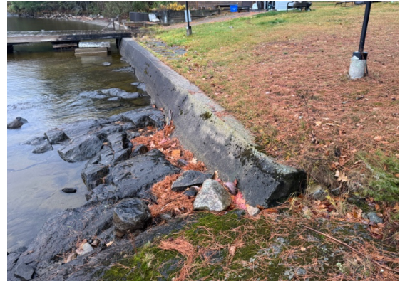
Photo 4. Breakwall on bedrock substrate
