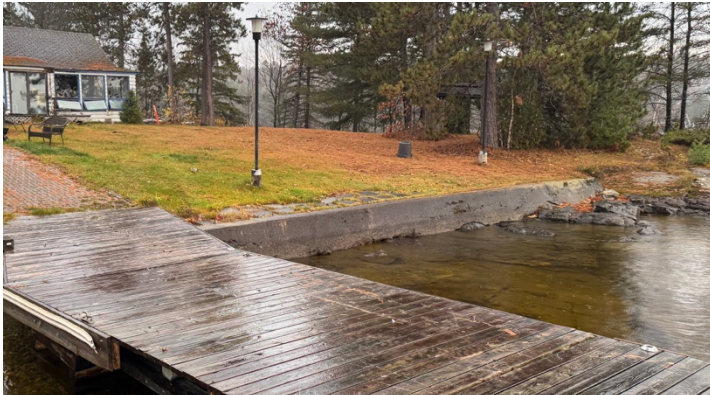
Photo 3. Dock and concrete breakwall on bedrock
