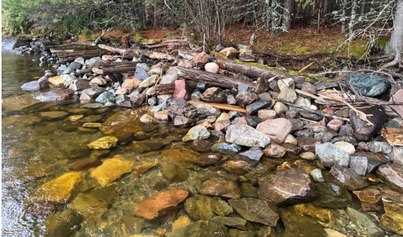
Photo 9. Boulder revetment that ties into bedrock shore at top left
