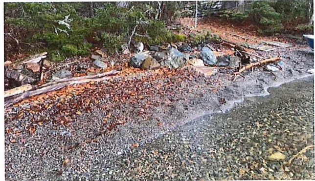
Photo 8. Boat launch, west side of this shore large section
