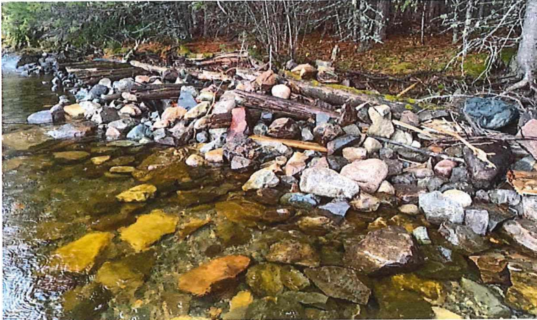
Photo 9. Boulder revetment that ties into bedrock shore at top left
