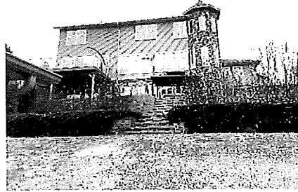
Figure 2: Image of rear of property looking south
