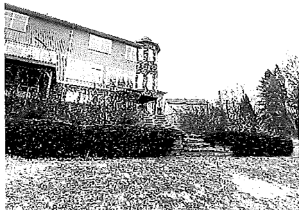
Figure 3: Image of rear of property looking west
