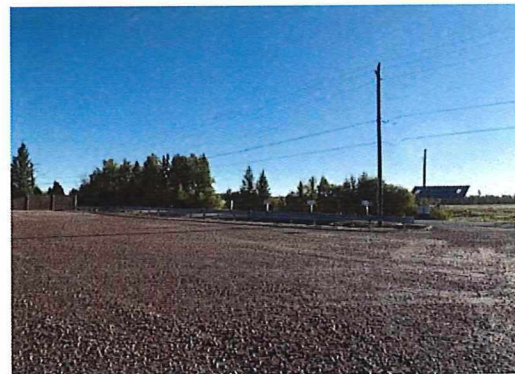
Figure 9: Vermillion Lake Road and Solar Panels, facing north-east from subject lands
