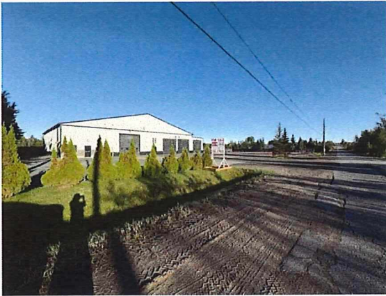
Figure 1: Photo of Building facing north-west
