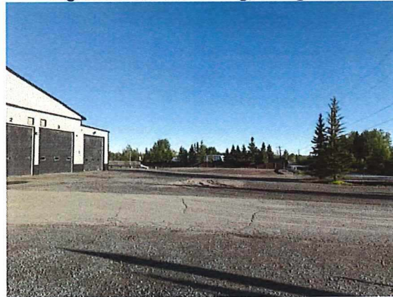
Figure 4: Photo of yard facing north
