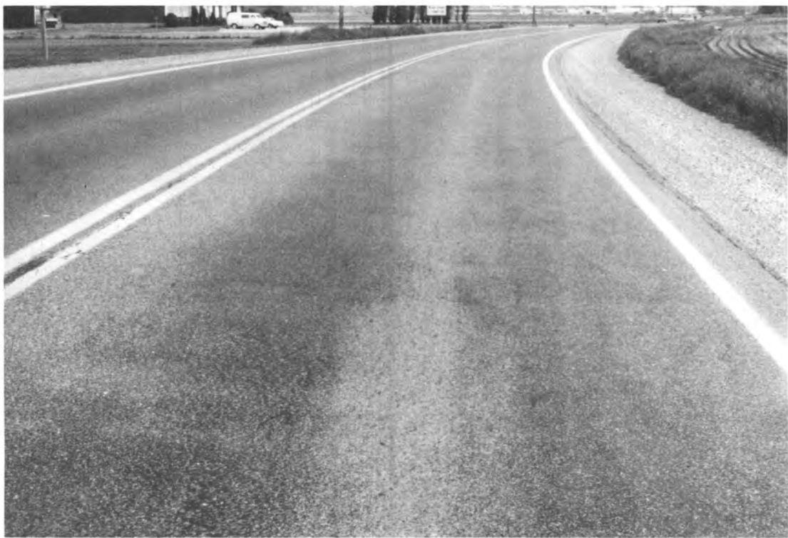
Moderate Flushing
