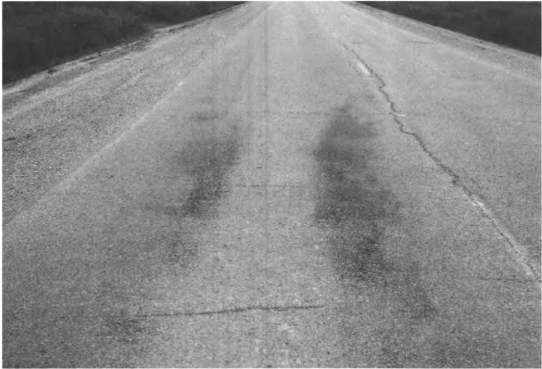
Slight Flushing
