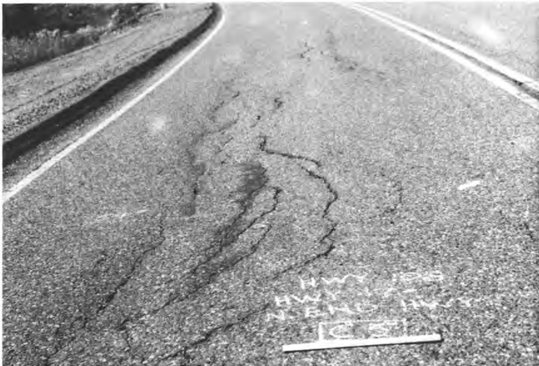
Slippage Crack
