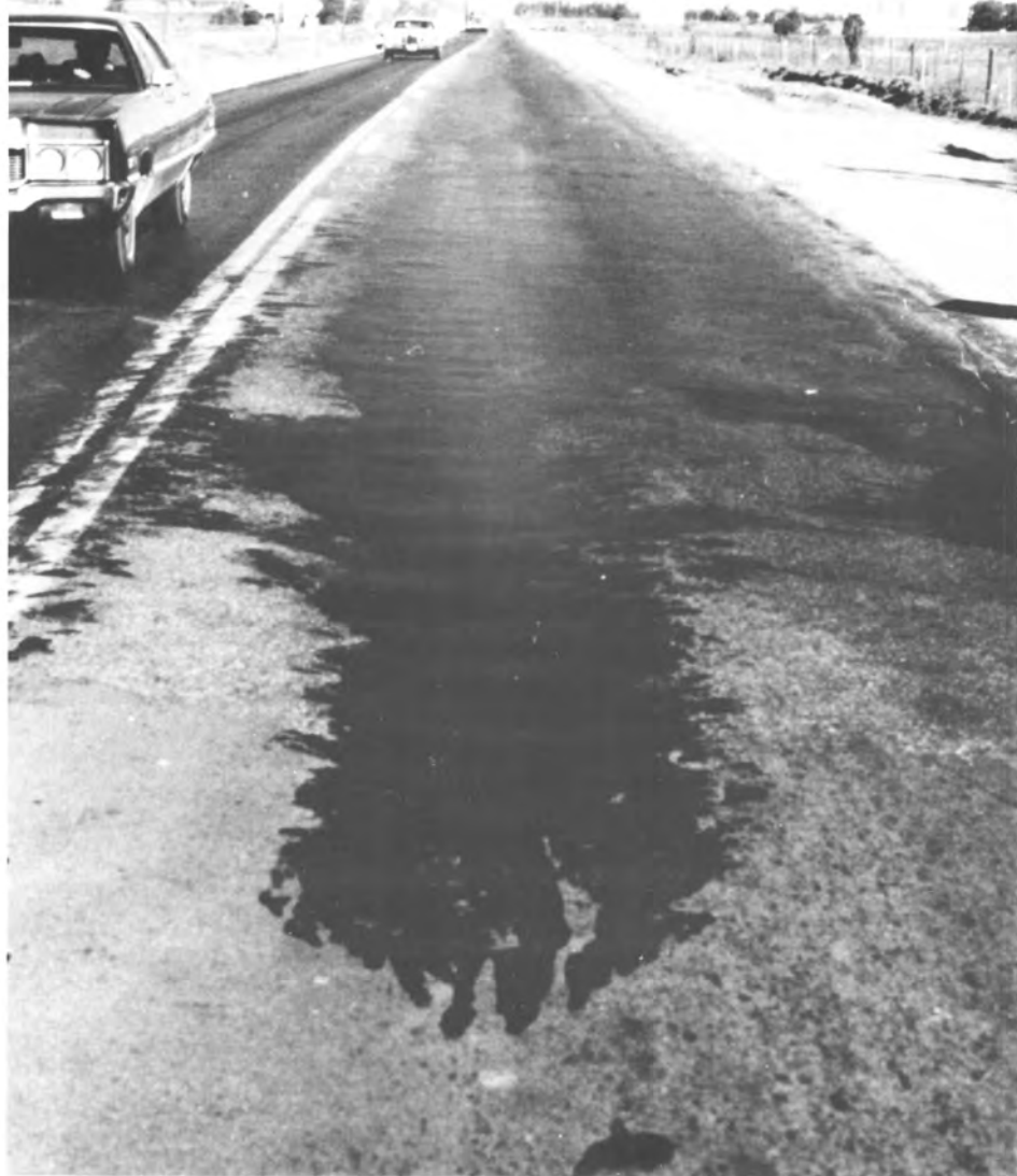
Very Severe Flushing
