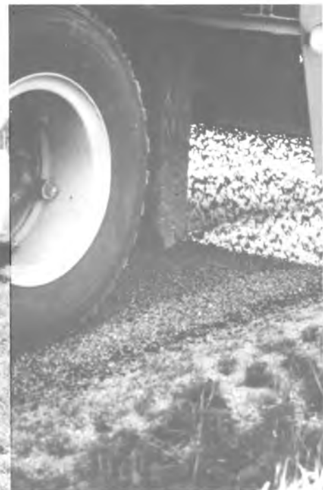
Machine Chip Seal Operation
