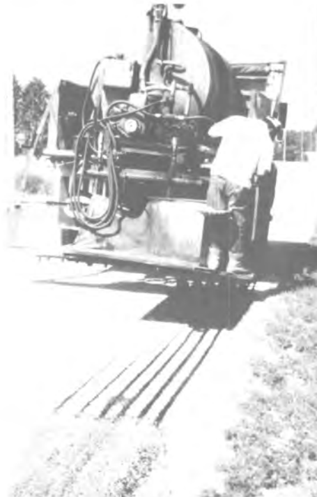
Machine Chip Seal Operation
