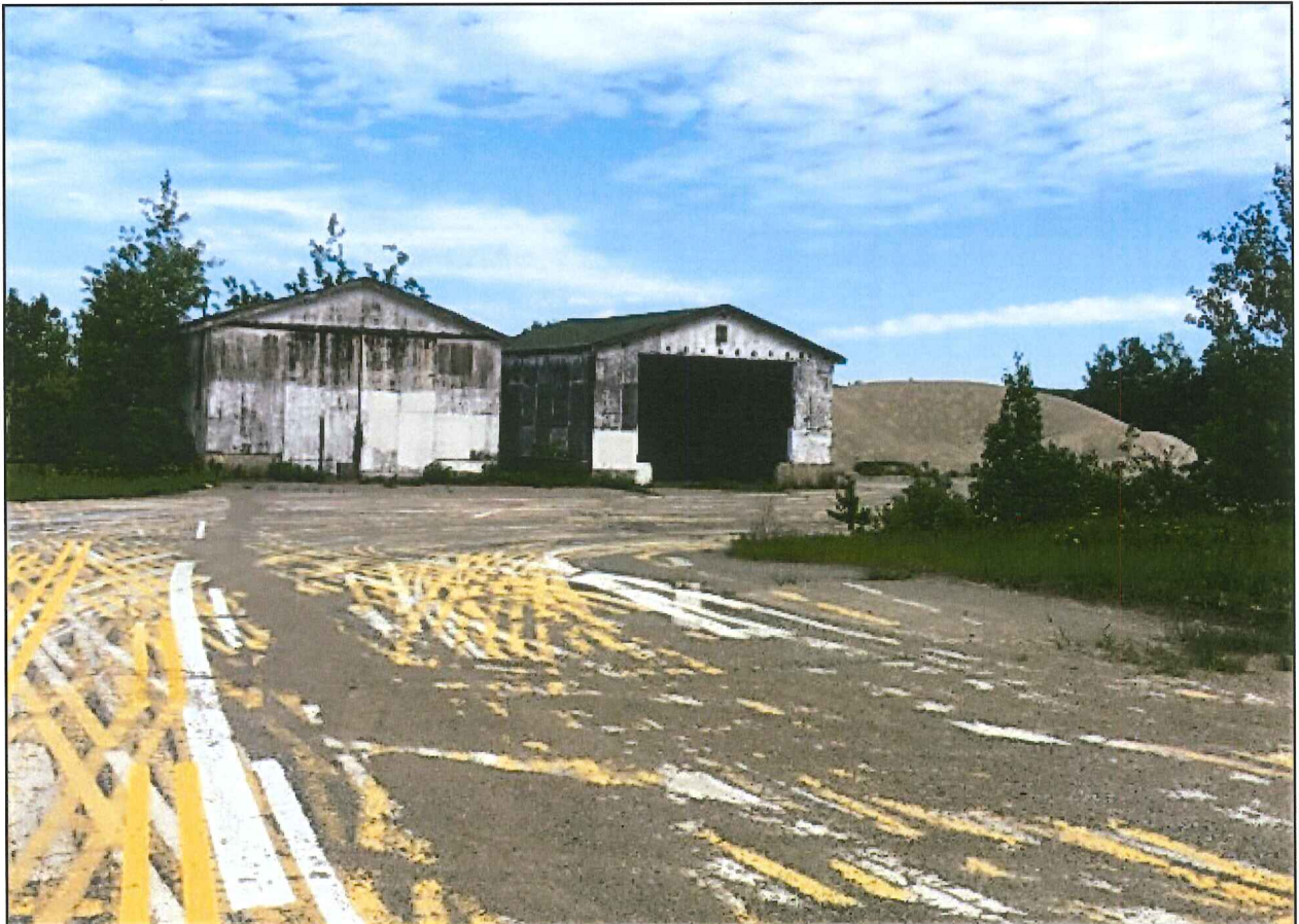
Former Sand/Salt Sheds
