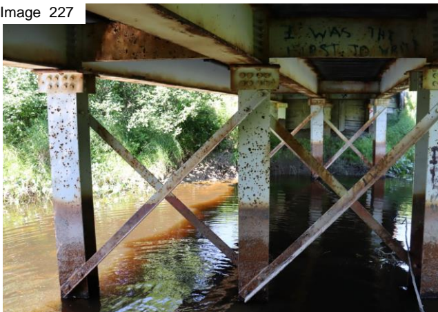
South pier pile perforation
