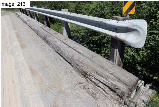
South deck surface damaged boards
