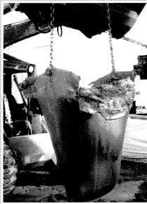
Silt Sack is a sediment control device used to prevent silt and sediment from entering your drainage system by catching the silt and sediment while allowing water to pass through freely. Siltsack can be used as a primary or secondary sediment control device to prevent failure of your drainage system due to clogging. It must be maintained on a regular basis to function properly. Silt sack is available in both high-flow or regular flow.
