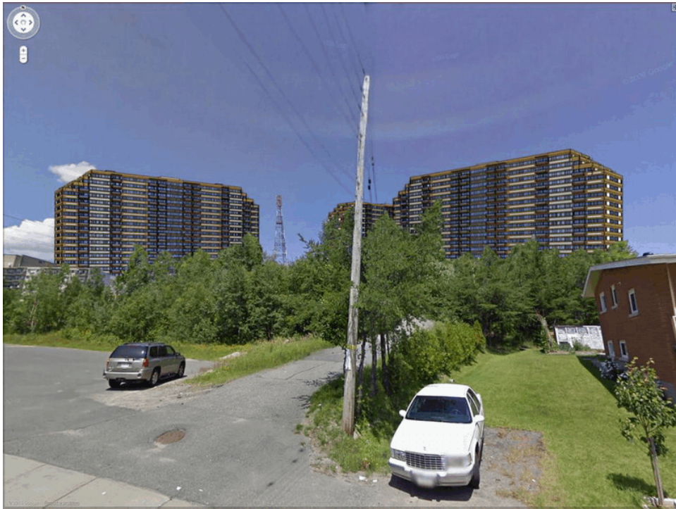
PERSPECTIVE 5 VIEW OF SITE LOOKING NORTH FROM WOOD AND VAN HORNE STREETS
